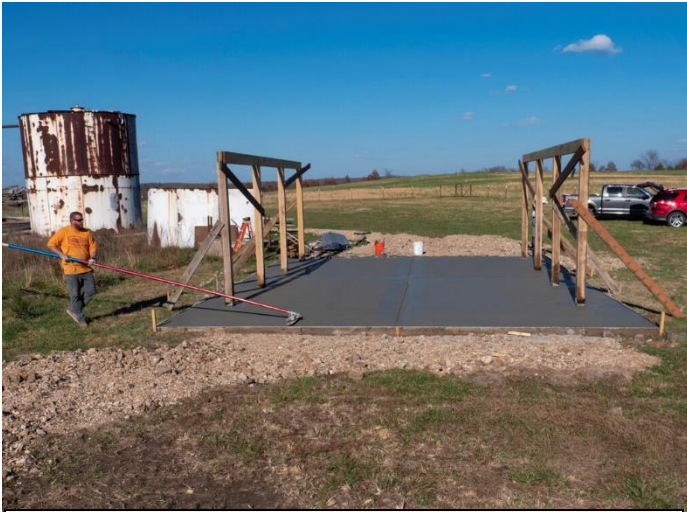
New concrete pad for the Pic Walenta Memorial Shelter
